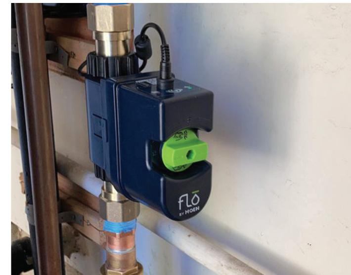
Commando Plumbing installed this smart water meter in a customer's home.
